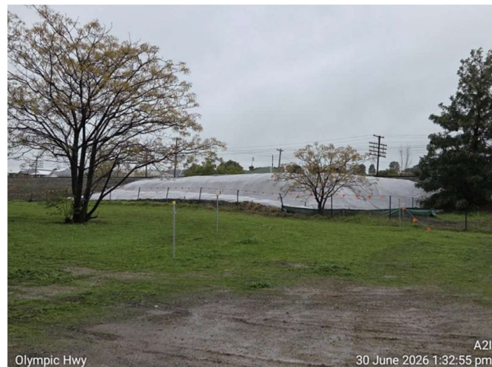
Figure 8. Junee Olympic Highway –stockpile covered with signage and flagging (30/06/26)
