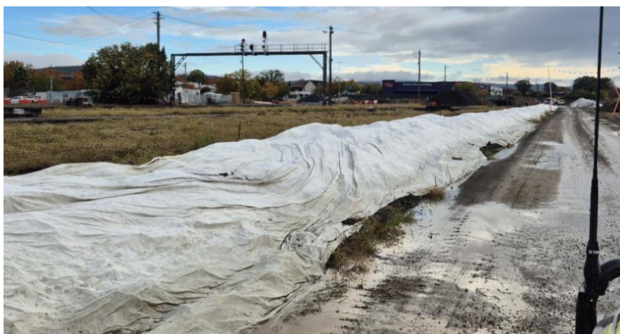
Figure 2. Albury Yard – protected stockpiles (19/05/26)
