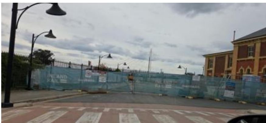
Figure 1. Albury Station – clean construction exit (03/05/26)
