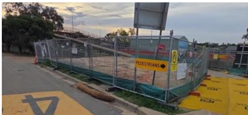
Figure 6. Cassidy St – erosion and sediment controls in place (03/05/26)
