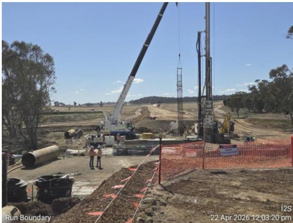
Figure 5. Run Boundary Creek – piling (22/04/26)
