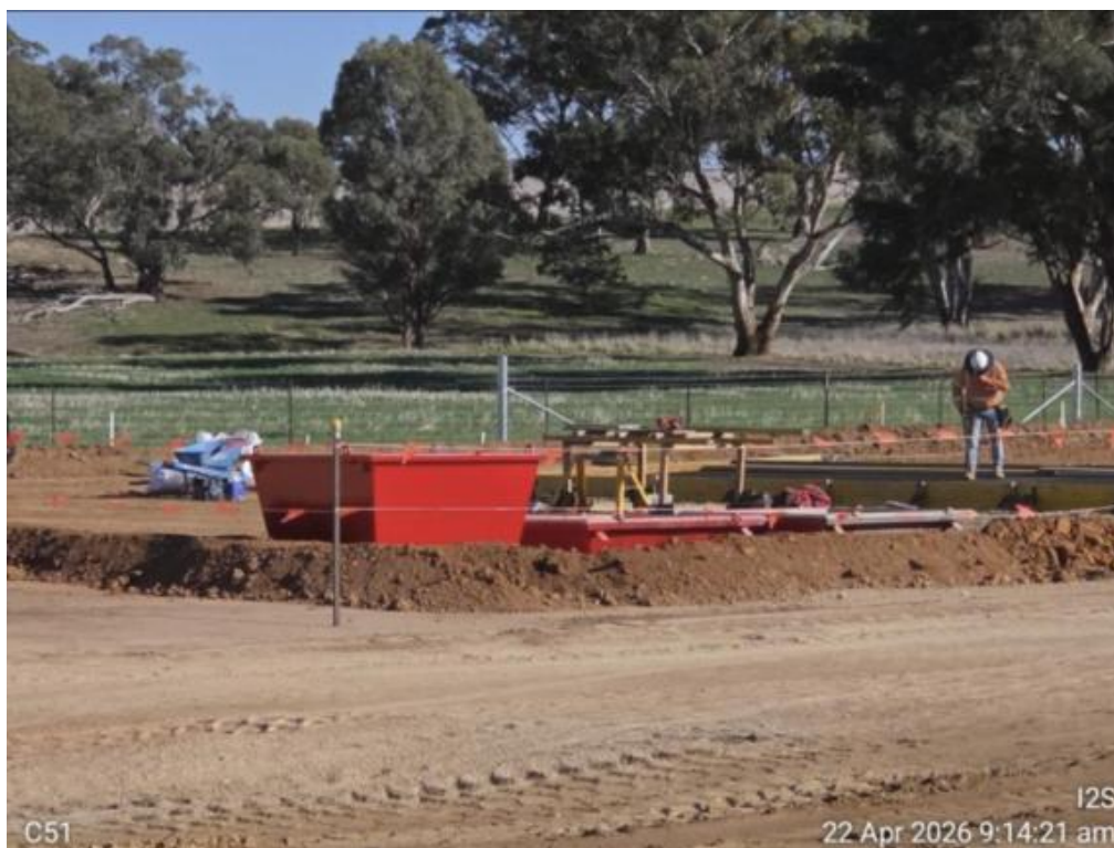
Figure 6. Cut 51 – use of waste receptacles, including steel concrete washout bins to enable concrete recycling (22/04/26)
