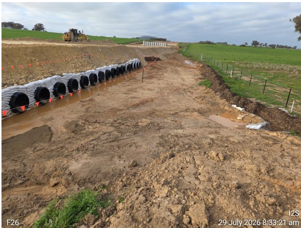
Figure 3. Sediment control – Fill 26 (29/07/26)
