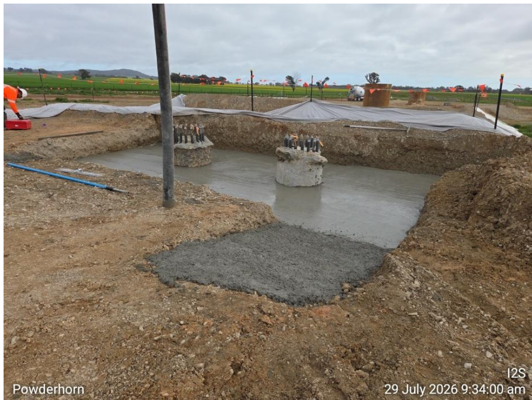
Figure 4. Piling works – Powderhorn Creek (29/07/26)
