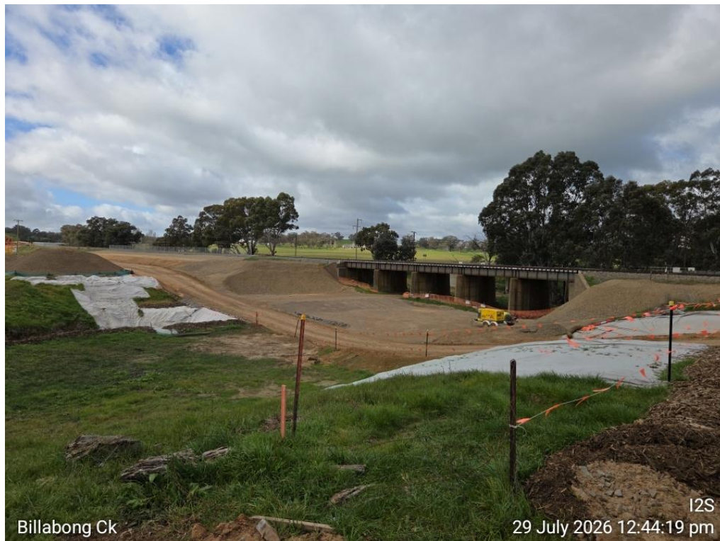
Figure 1. Billabong Creek construction crossing (29/07/26)
