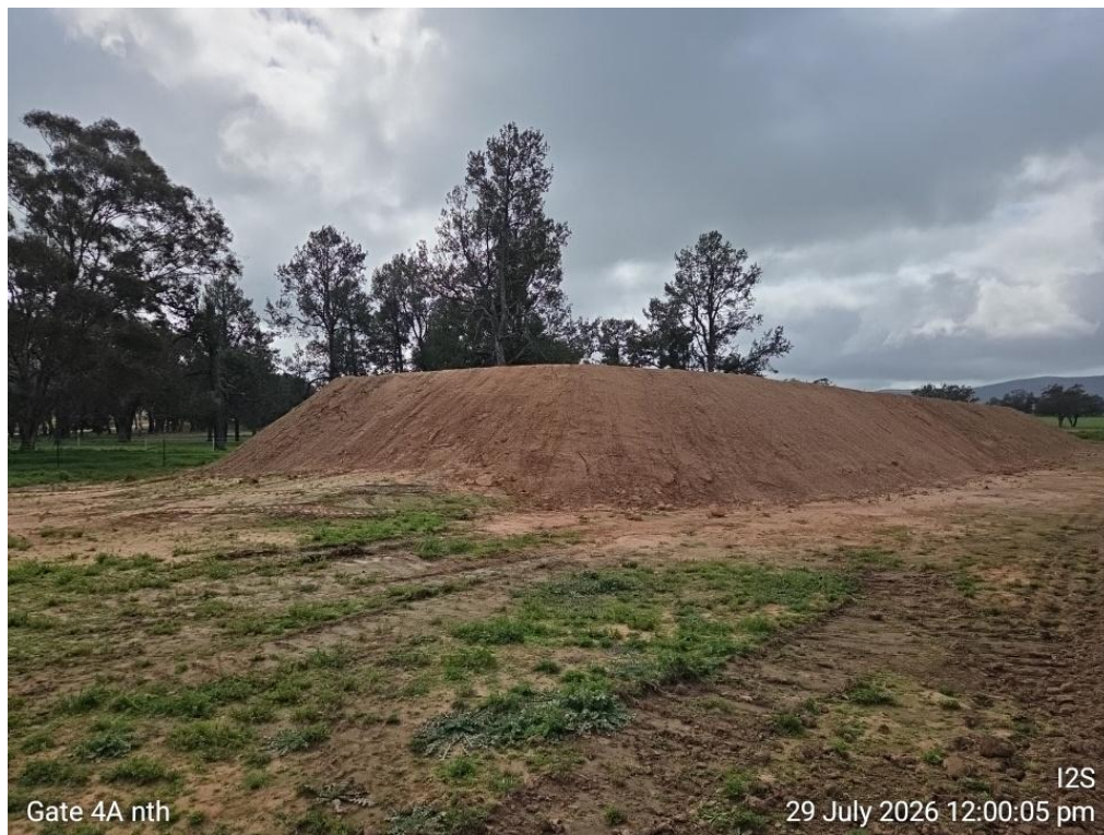
Figure 2. Gate 4A stockpile awaiting soil binder protection (29/07/26)
