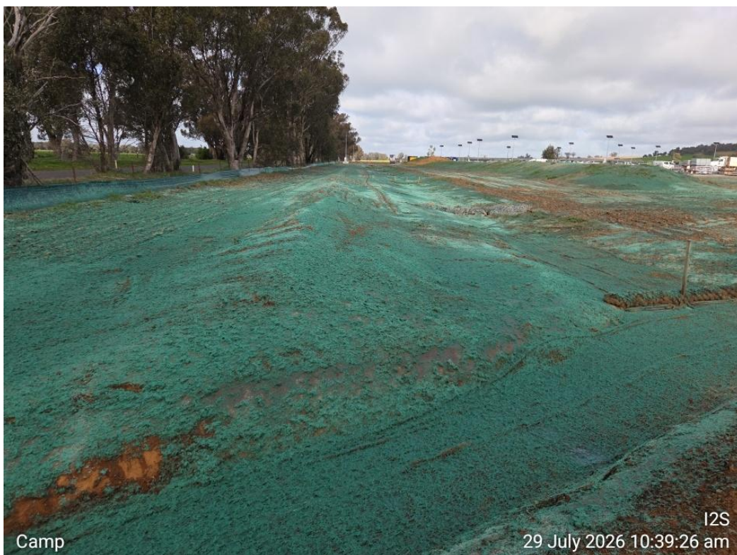
Figure 5. Stockinbingal Accommodation Camp – recent hydromulching (29/07/26)
