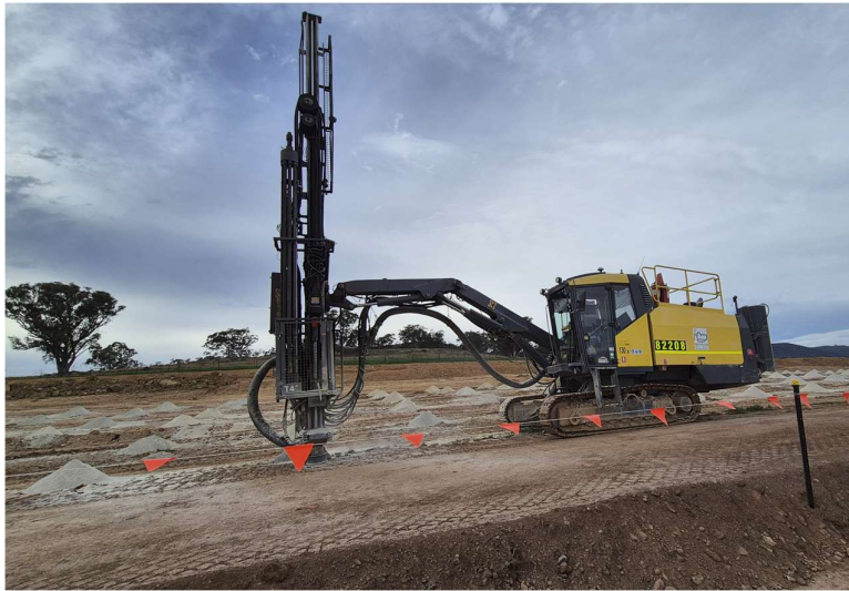
Figure 5. Corridor –Blasting preparatory works (17/06/26)
