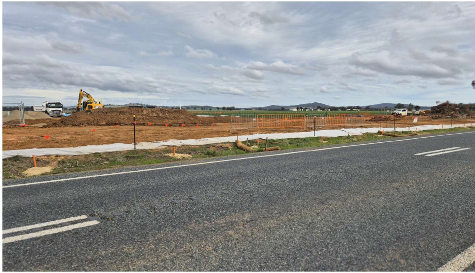
Figure 4. Burley Griffin Way –Geofab along batter, coir logs along swale (17/06/26)
