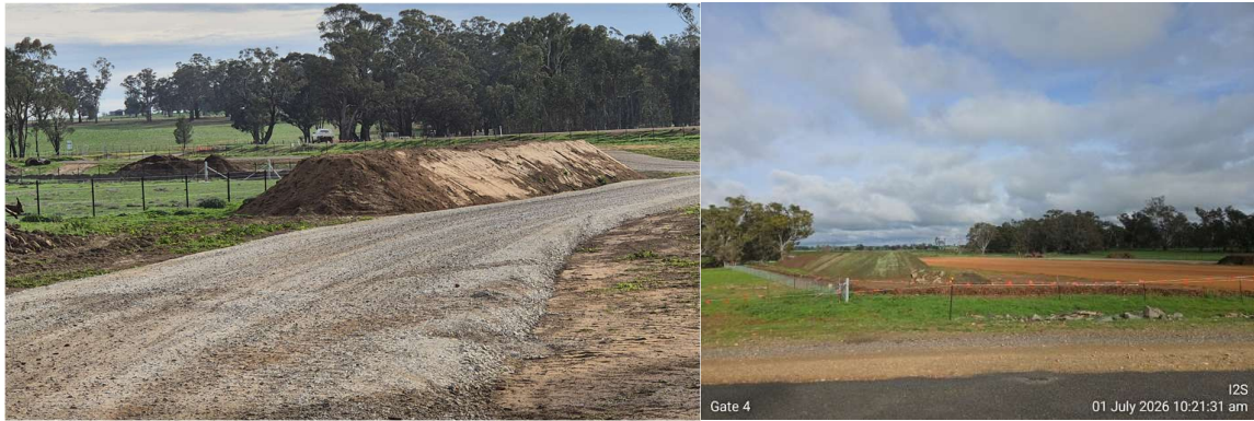
Figure 3. Ullandra Creek - stockpiles unprotected (17/06/26 left) – Binder applied in stockpiles (01/07/26 right)
