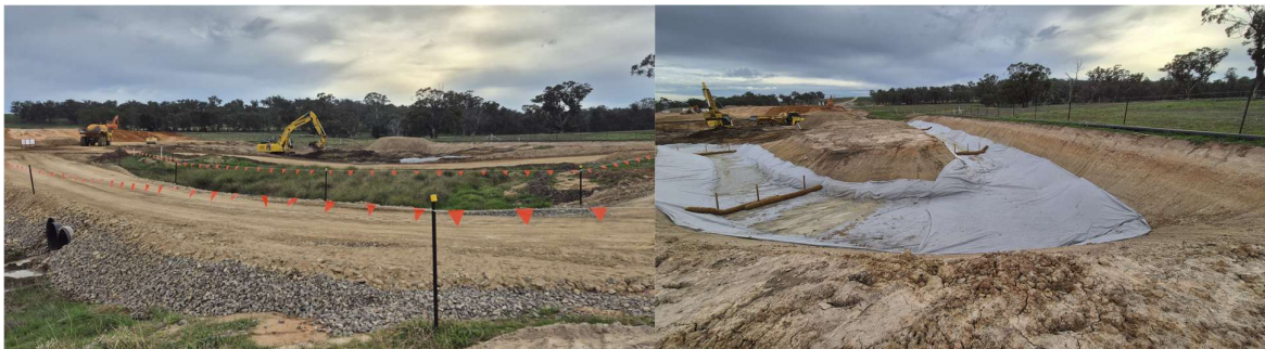
Figure 2. Dirnaseer Rd south –Diversion works in progress (17/06/26)
