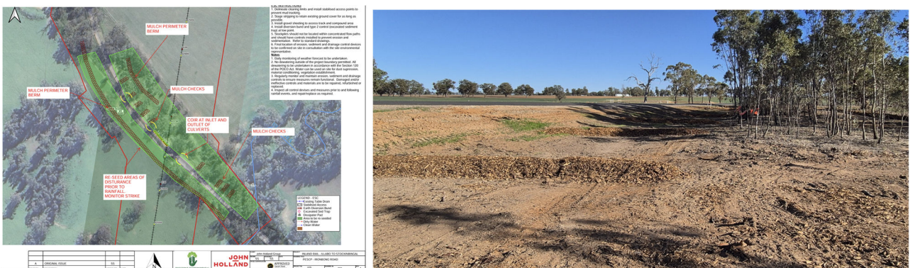
Figure 3. Ironbong Rd Progressive ESCP prepared and to be certified by CPESC (JHG, 2/04/26 left) (ER inspection 25/03/26 right, soils to be stabilised)
