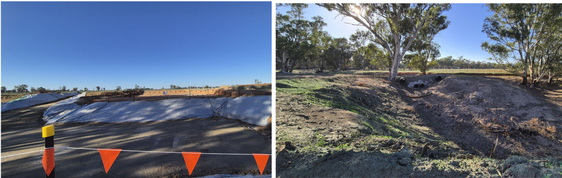
Figure 4. Ullandra Creek (ER inspection 25/03/26)- temporary bund along front edge of pad to be installed in accordance with CPESC report dated 6/03/26
