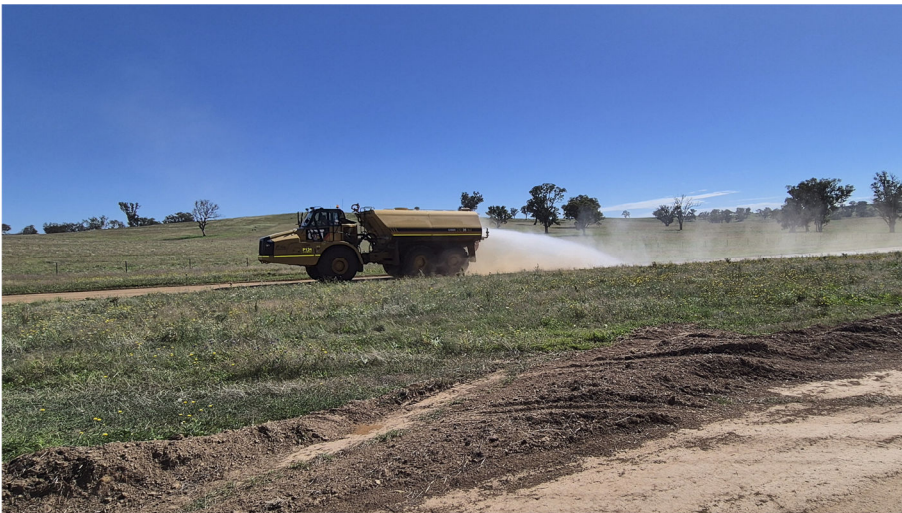
Figure 5. Water cart use along corridor (ER inspection 25/03/26)
