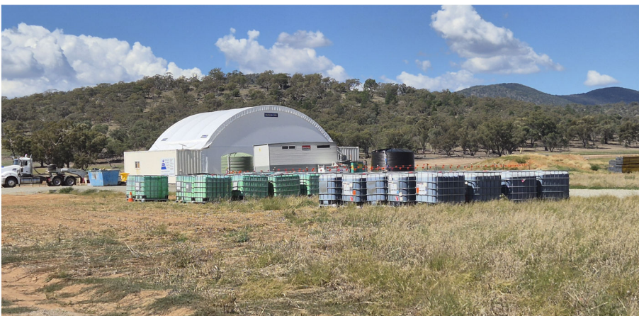
Figure 6. Soil Binder storages in Dirnaseer Rd compound – Brown containers: haul roads binder, Green containers: spoil (ER inspection 25/03/26)
