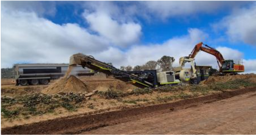
Figure 3. Corridor – crusher in operation (20/05/26)
