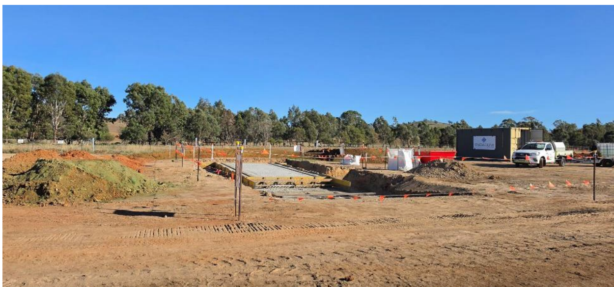
Concrete pad works in progress with concrete waste bin available.
