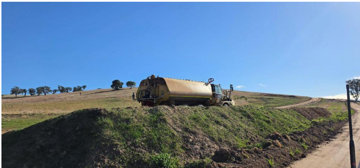
Water cart available on site.
