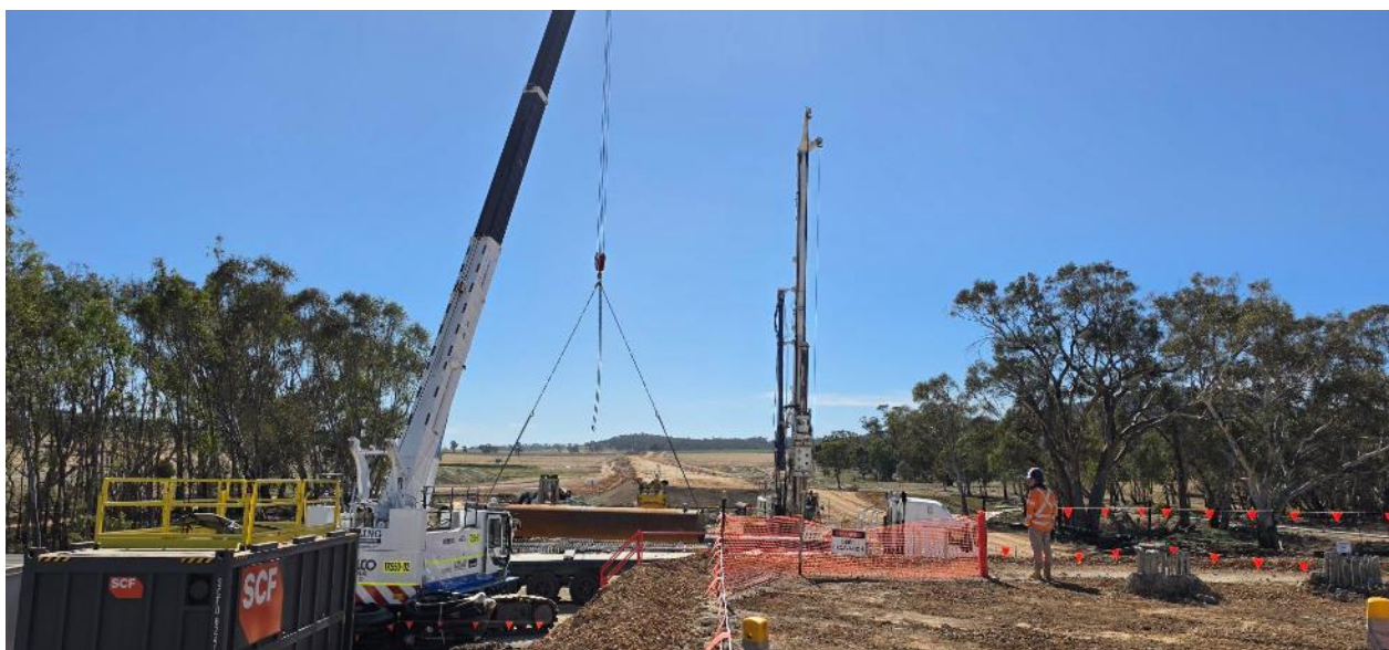
Piling works in progress at Run Boundary Creek.
