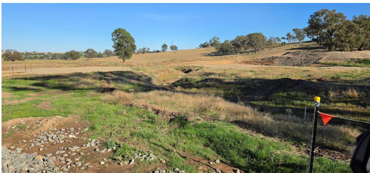
Mulch used in some areas for erosion and sediment control.
