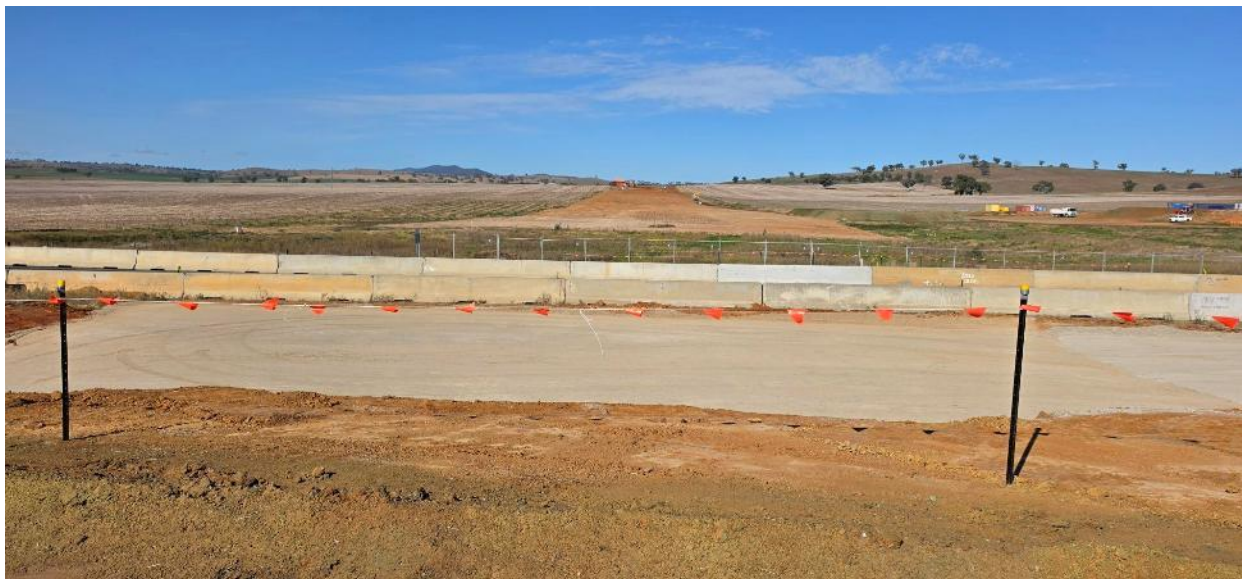
Piling Pad installed at Dirnaseer Rd.
