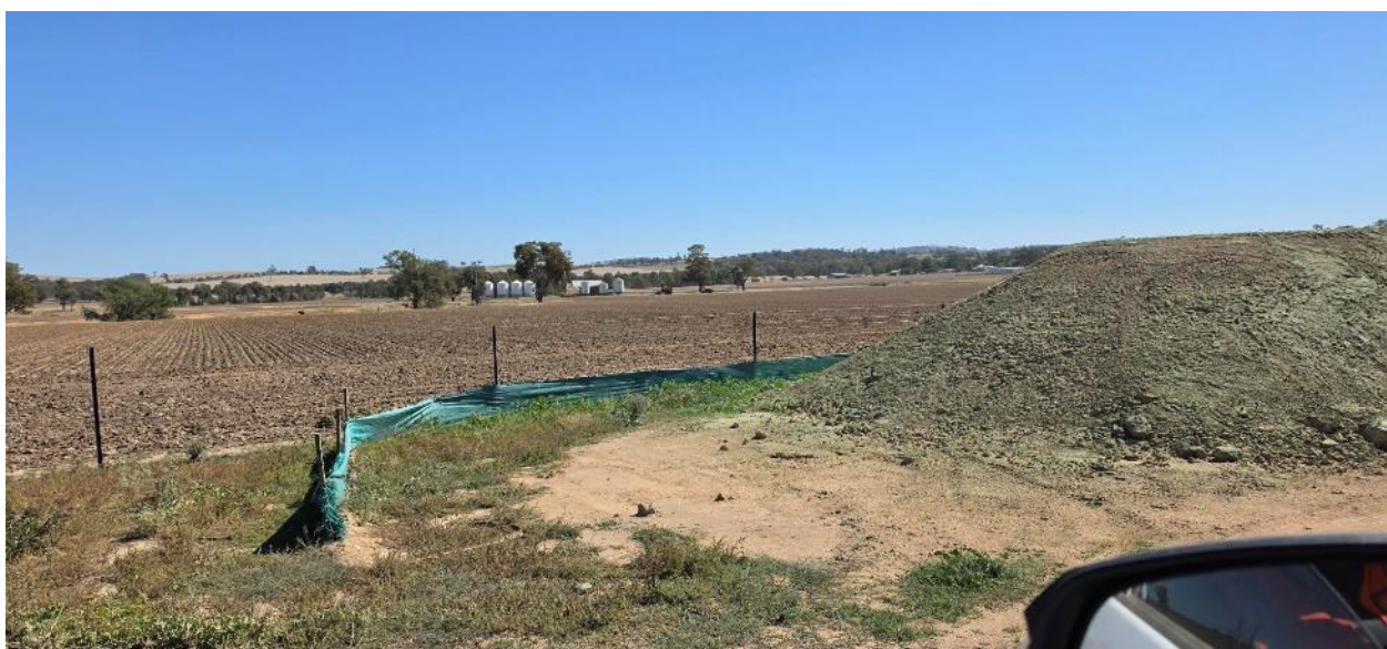
Sediment fence installed around stockpile. Stockpile sprayed with polymer for dust suppression.
