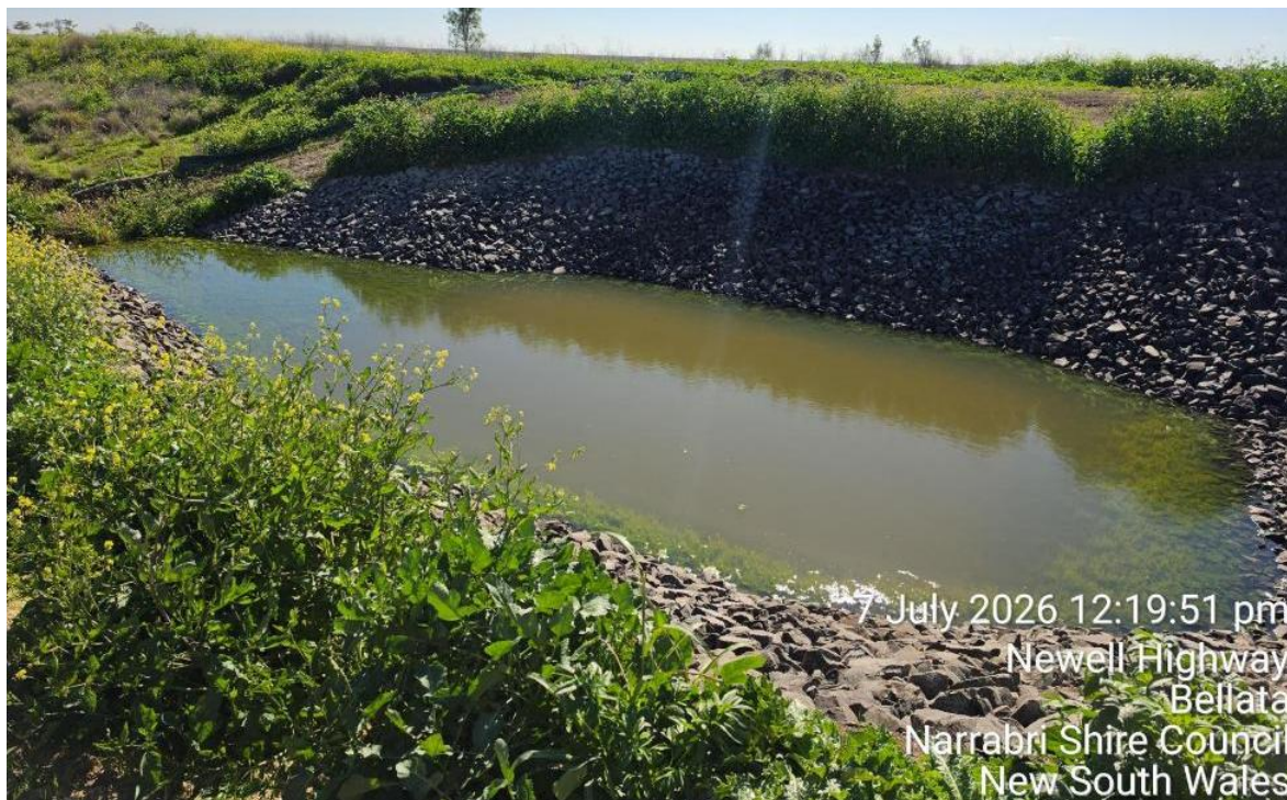
Rock lined basin downstream of the culvert, with vegetation evident above batters and in swale
