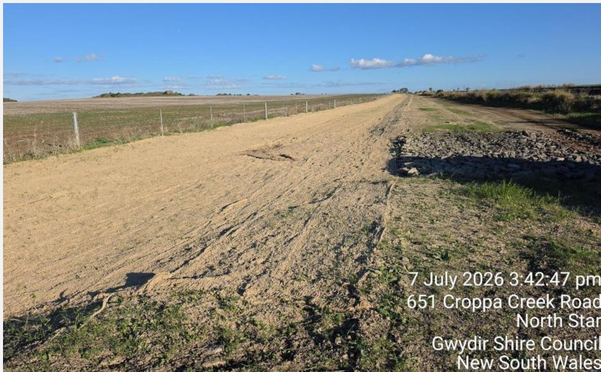
Rehabilitated swale drain and associated rock mattress adjacent to LX3166.
