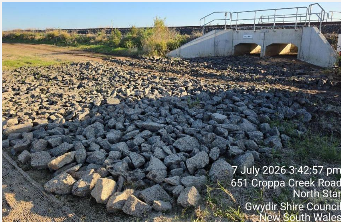
Existing culvert crossing with rock armouring as part of the rectification works adjacent to LX3166.
