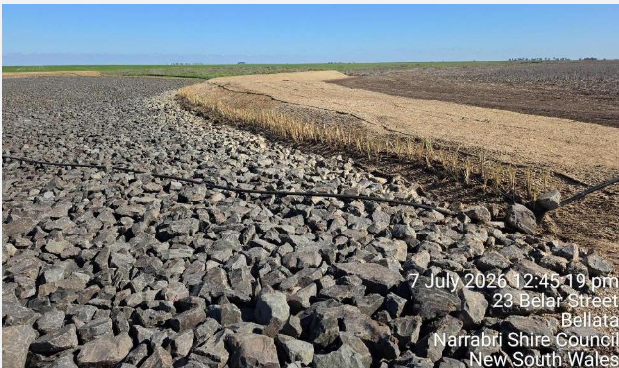
Rehabilitated batter stabilised with jute mesh and hydromulch.
