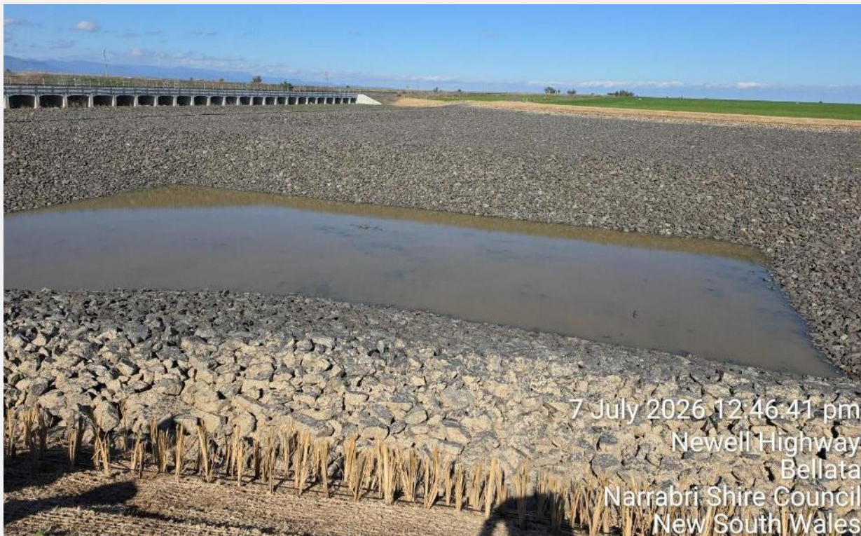
Rock-armoured basin within the reconstructed creek channel.
