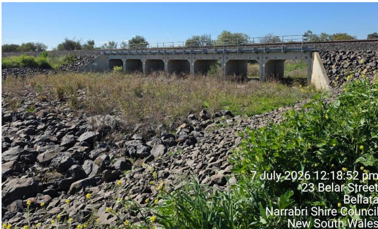
Downstream view of the culvert crossing showing rock mattresses in creek bed and behind head walls
