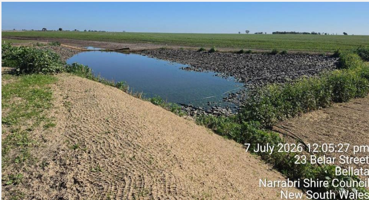
Rock-armoured basin within the reconstructed creek channel.
