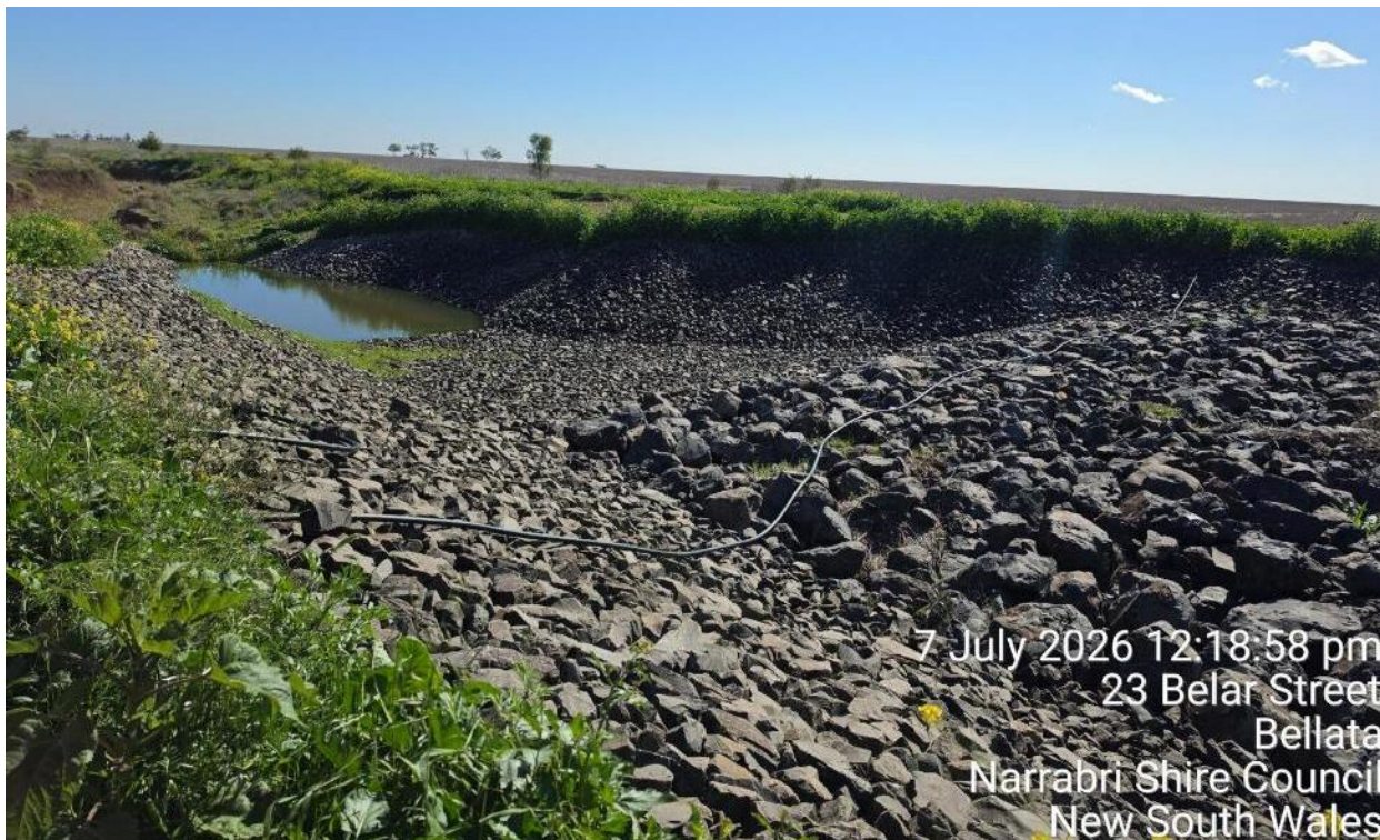
Downstream basin comprising riprap and vegetated swale
