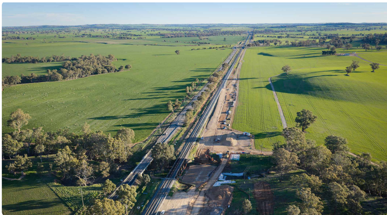
Image: Start of greenfield track (southern tie-in north of Illabo)
