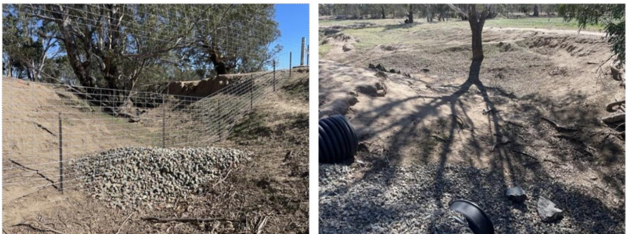
Figure B-6 Downstream and upstream (respectively) at Ulandra Creek – March 2026
