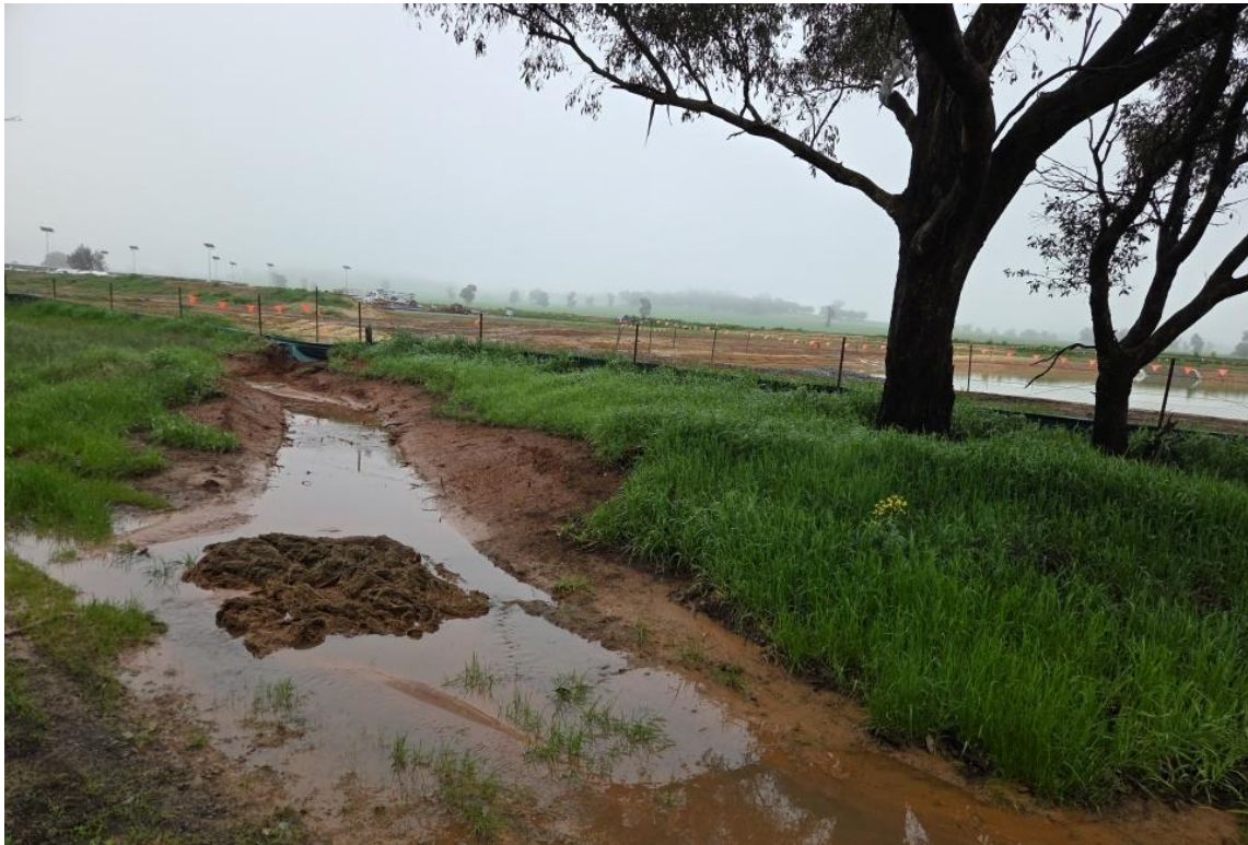
Figure 4. Stockinbingal Accommodation Camp - drainage stabilisation works to be undertaken (26/08/26)
