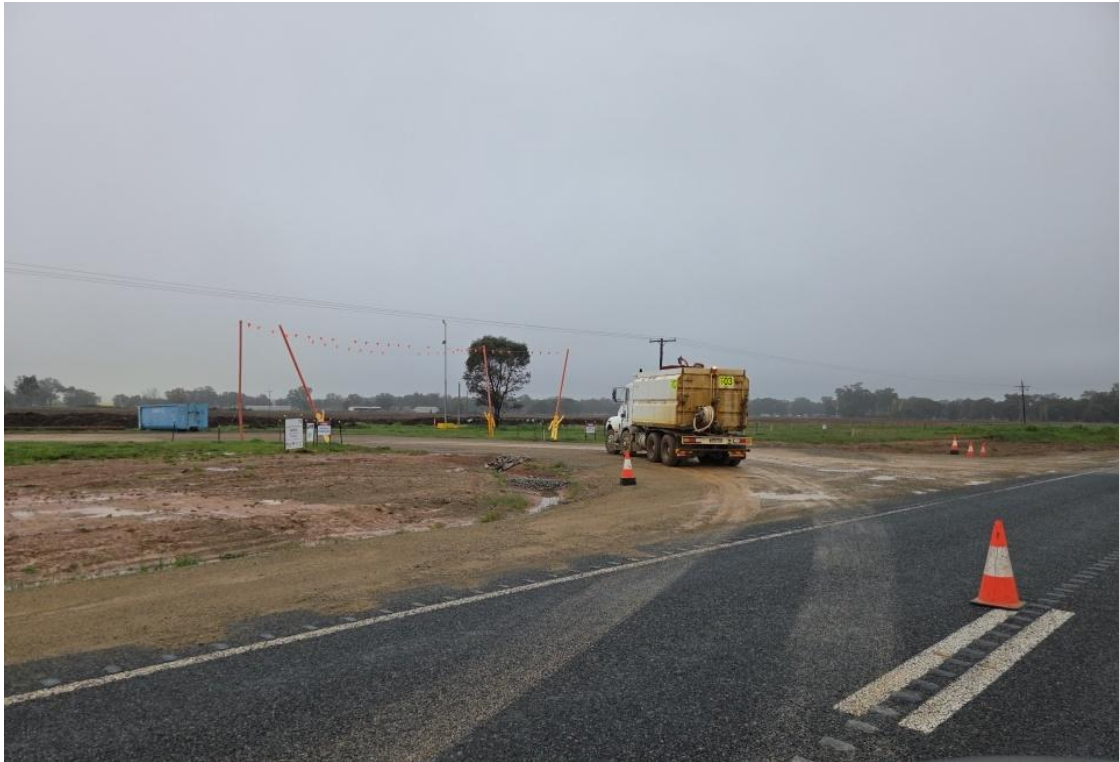
Figure 2. Burley Griffin Way – additional access stabilisation to be undertaken (26/08/26)
