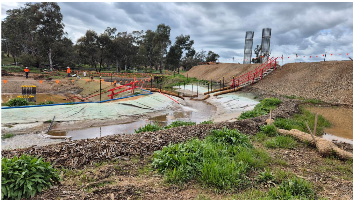
Figure 1. Isobel Creek clean water diversion and dewatering (12/08/26)
