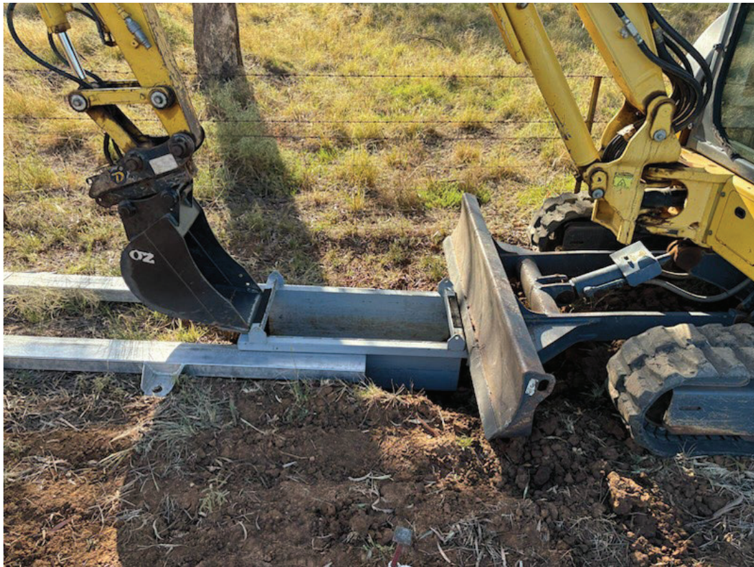
Figure 7: Sampling frame placed into access trench between the guide sleepers.
