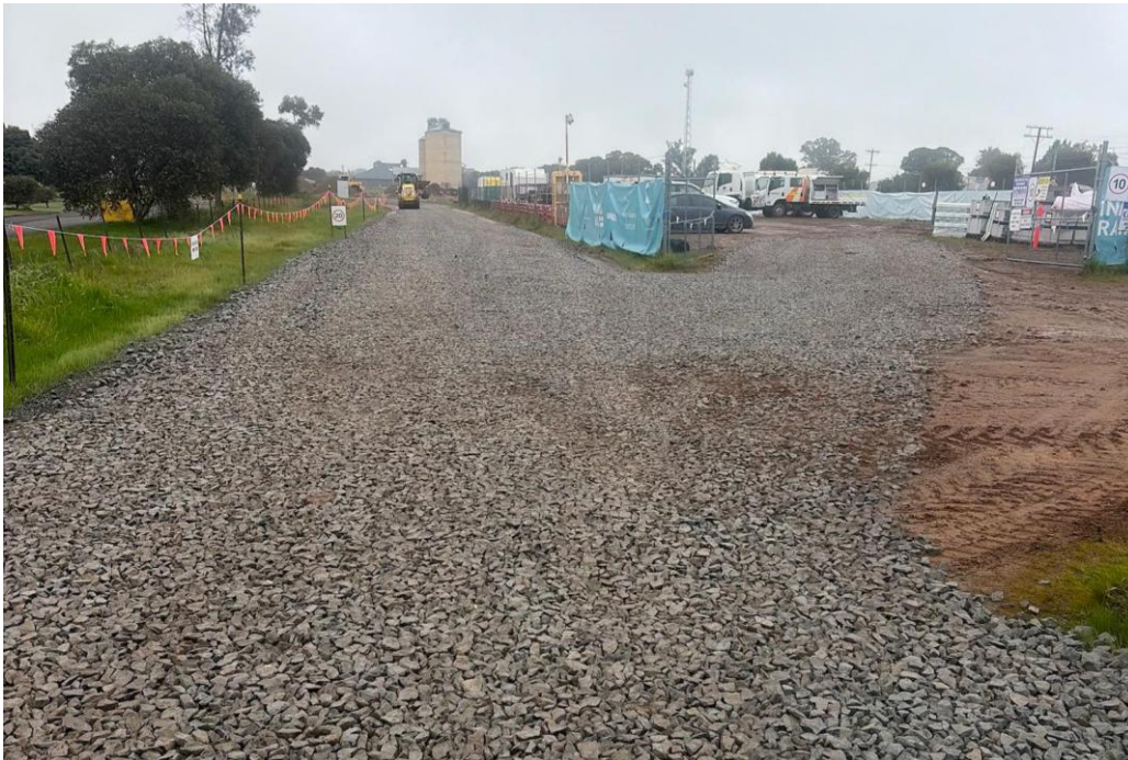
Figure 4. Yerong Creek – stabilised access (close-out of action) (26/08/26)
