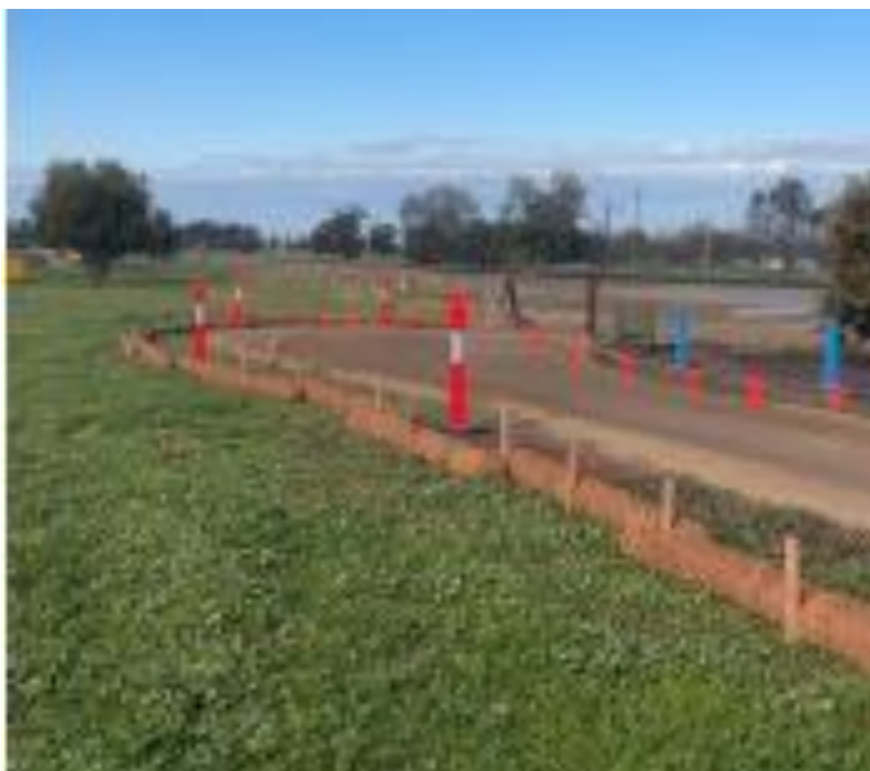
Figure 5. Yerong Creek – stabilised access (close-out of action) (31/08/26)
