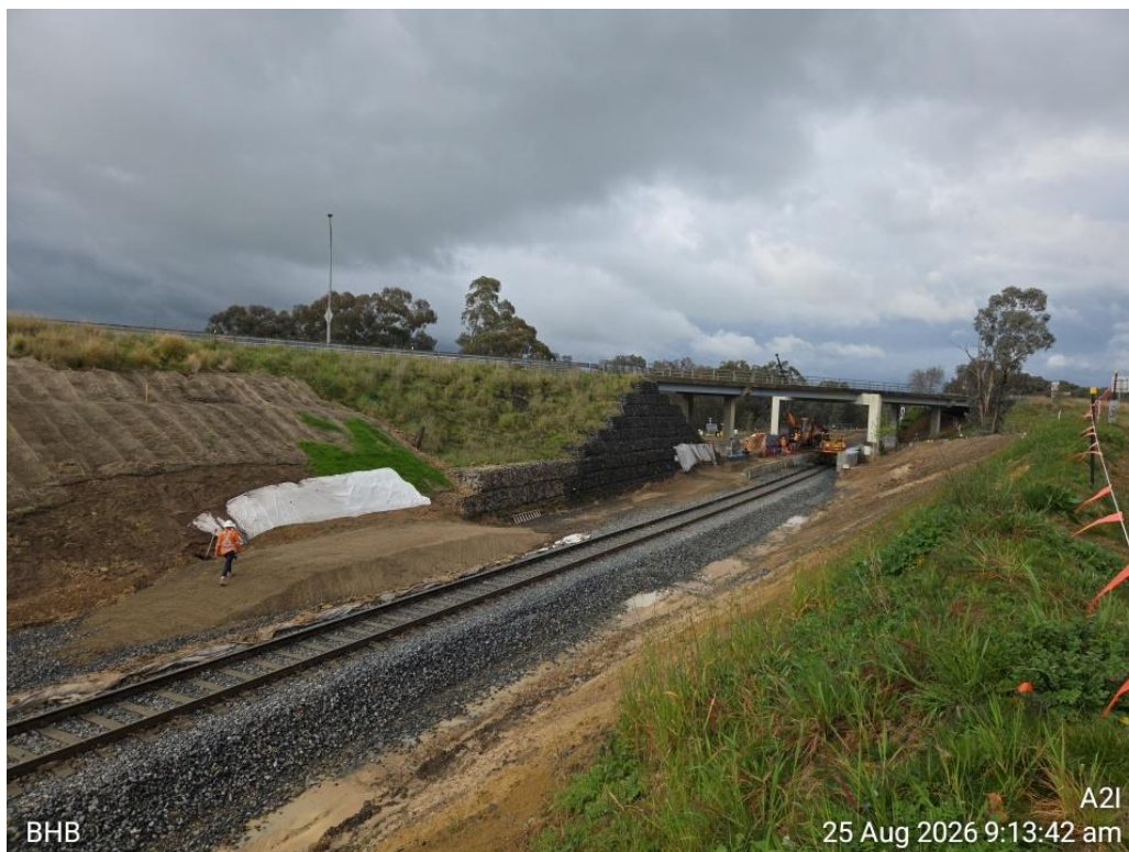
Figure 3. Billy Hughes Bridge – Progressive batter stabilisation (25/08/26)
