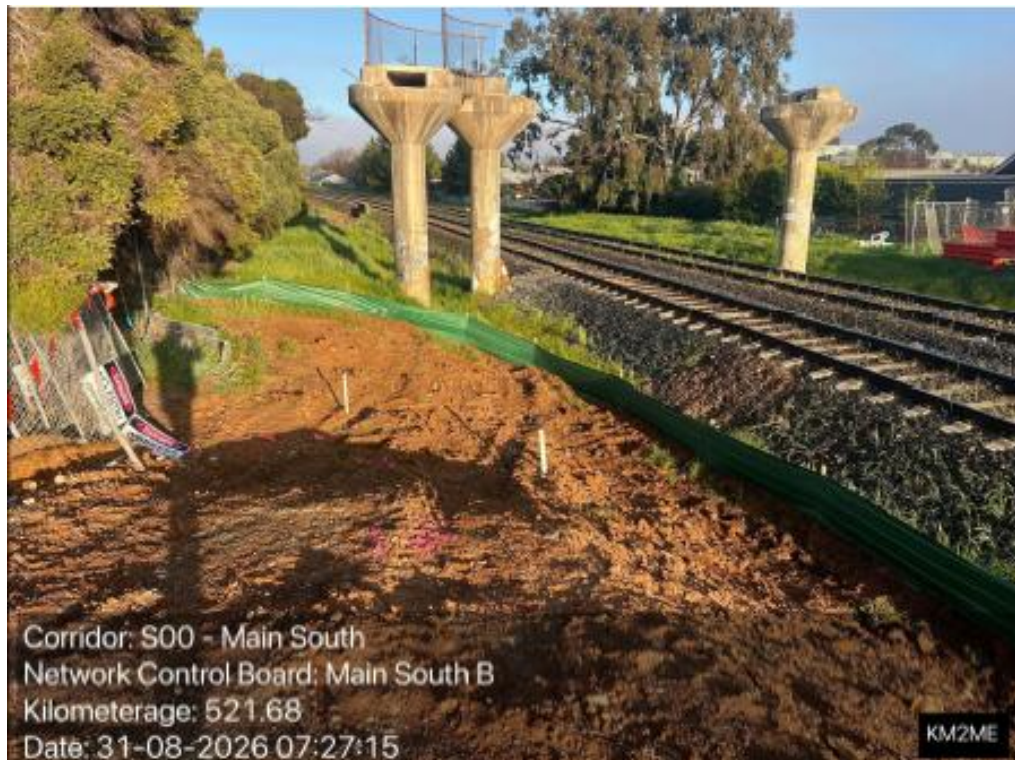
Figure 6. Cassidy – sediment fence installed (close-out of action) (31/08/26)
